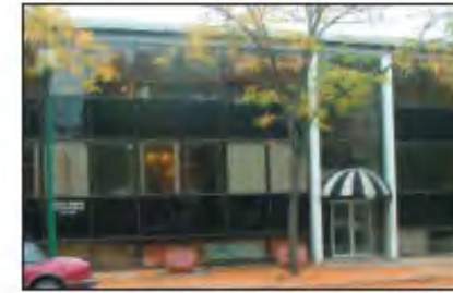
Building with no defined base, middle, or top. (4.7.2.1)
